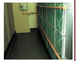
The VESDA by Xtralis air-sampling pipe network does not interfere with the fan filters or ongoing maintenance at the Wells Fargo Center in Minneapolis.
